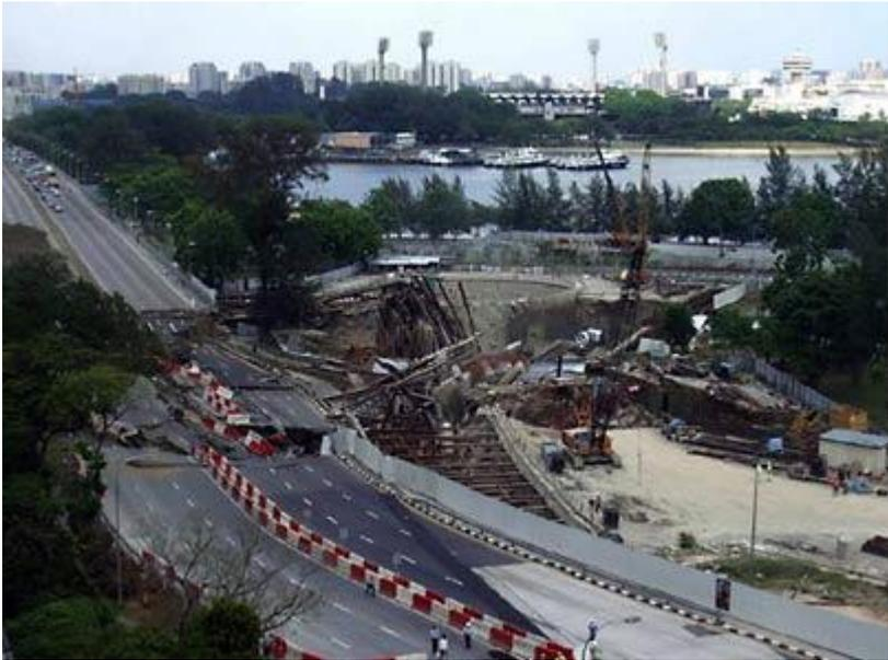
The original design misinterpreted the local geology and overestimated the soil shear strength in its analysis. (*Whittle, 2004*)
